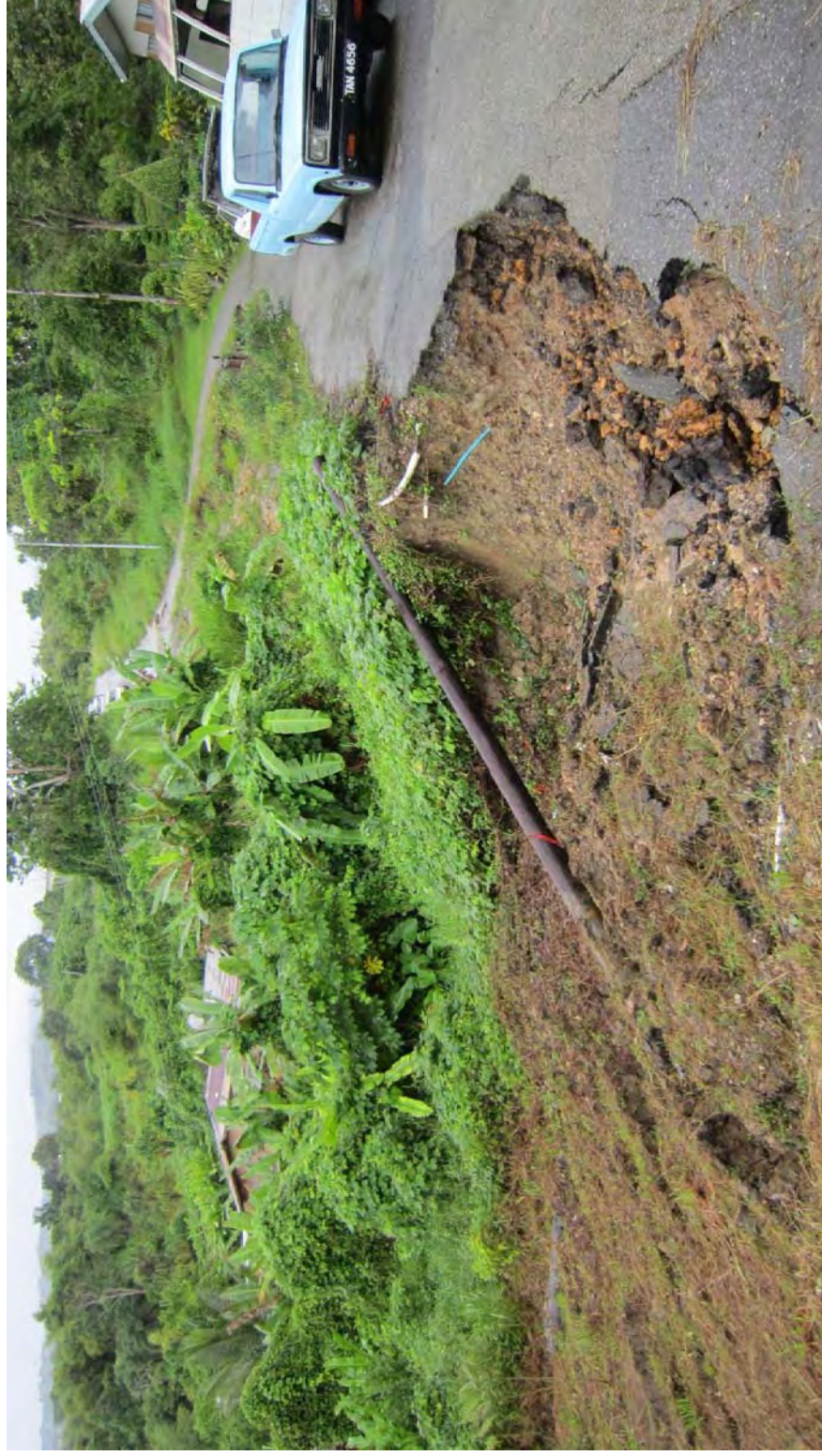
Figure 8.2 Typical Landslide Failure along Secondary Roads in Trinidad caused by leaking water mains.
