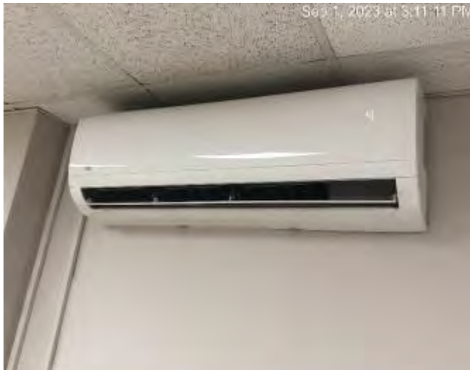
Tempblue 2 Ton Split Unit located in ground floor reception area.
