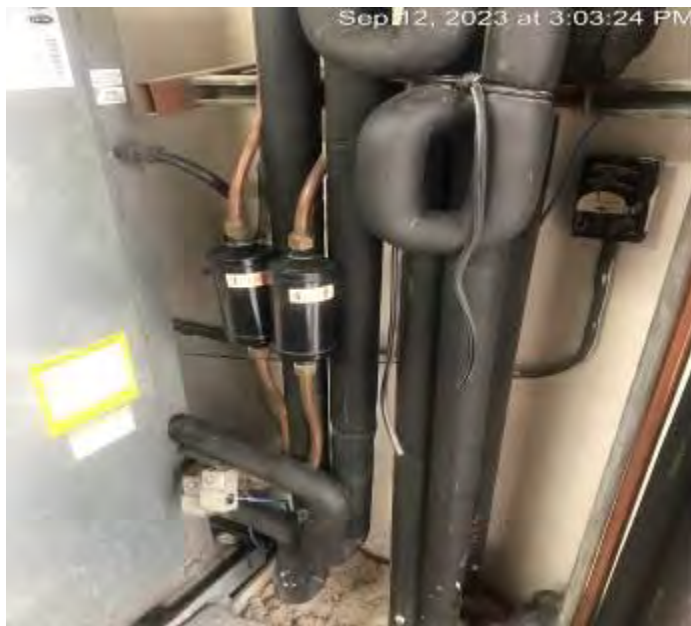
Carrier Air Handler Unit dual coil piping set up
