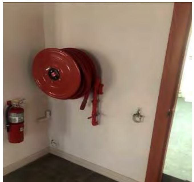
Typical Fire Hose Reel and Fire Extinguisher
