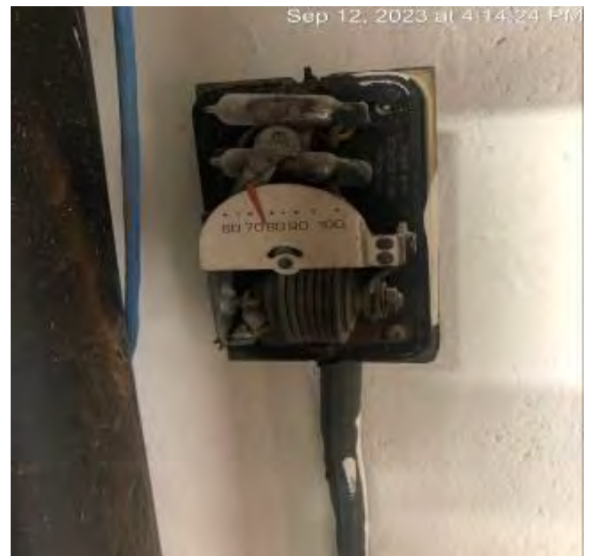
Air Handler Unit old Thermostat connection to unit. Digital Thermostat installed in room but connection to unit cannot be traced
