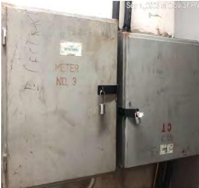
T&TEC C.T and Meter Cabinets
