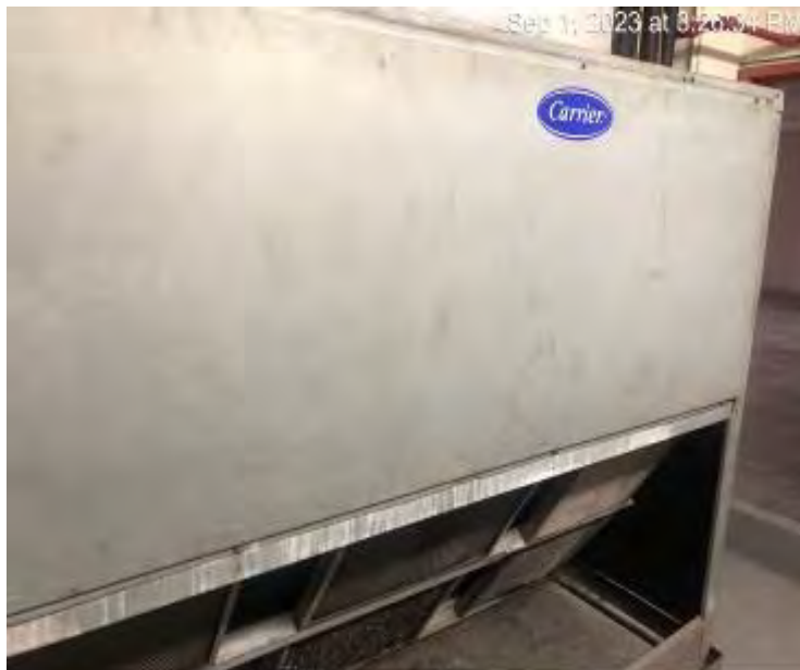
Carrier Air Handler Unit with non-MERV rated filters installed
