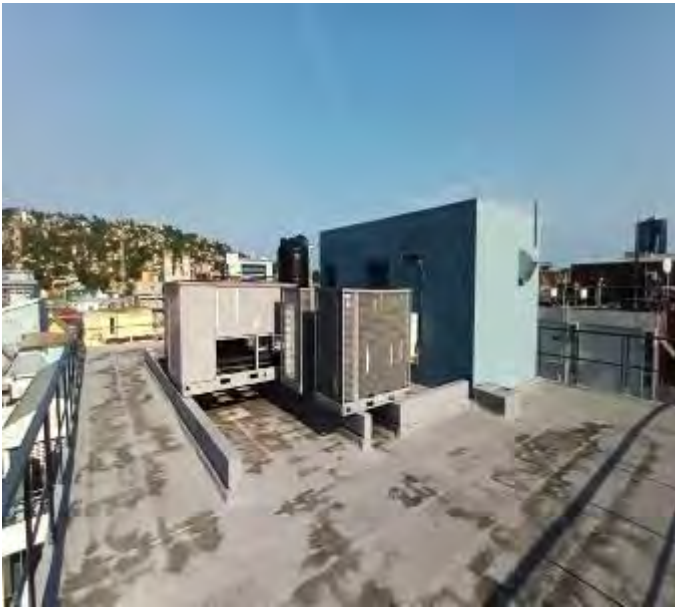
Air Conditioning Condensers located on Roof Level
