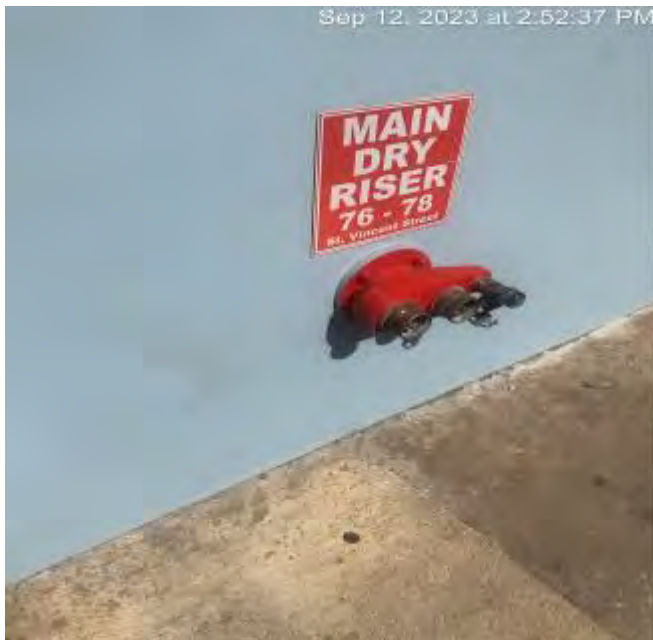
Building Main Fire Dry Riser
