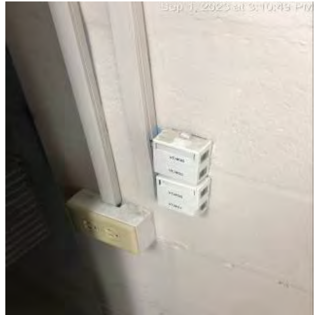
Typical Voice/Data Outlet on Ground Floor
