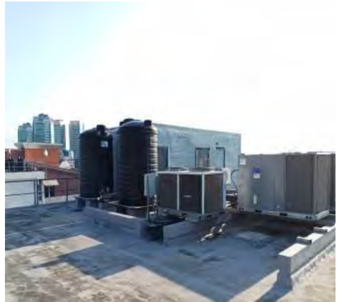
Air Conditioning Condensers located on Roof Level
