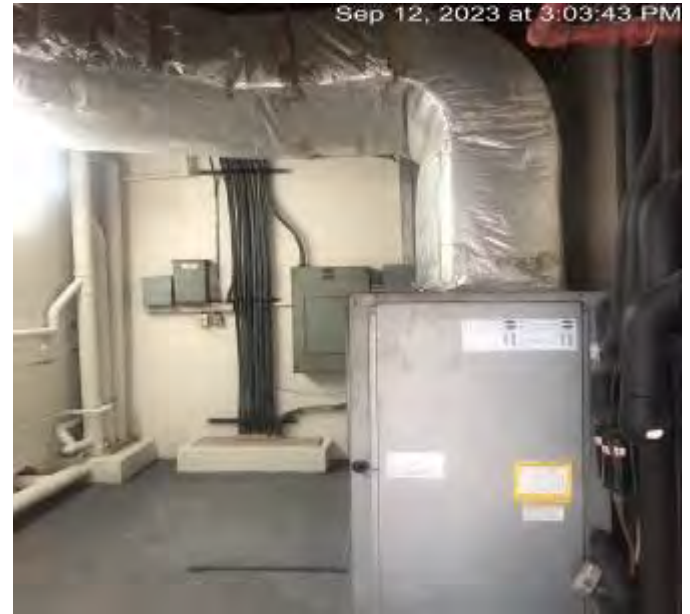
Carrier Air Handler Unit set up
