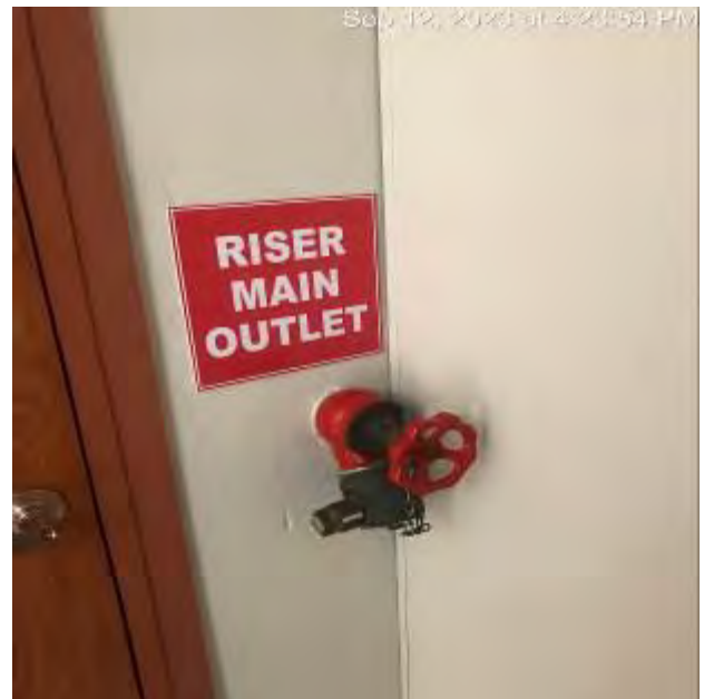
Building Main Riser Outlet located on each floor
