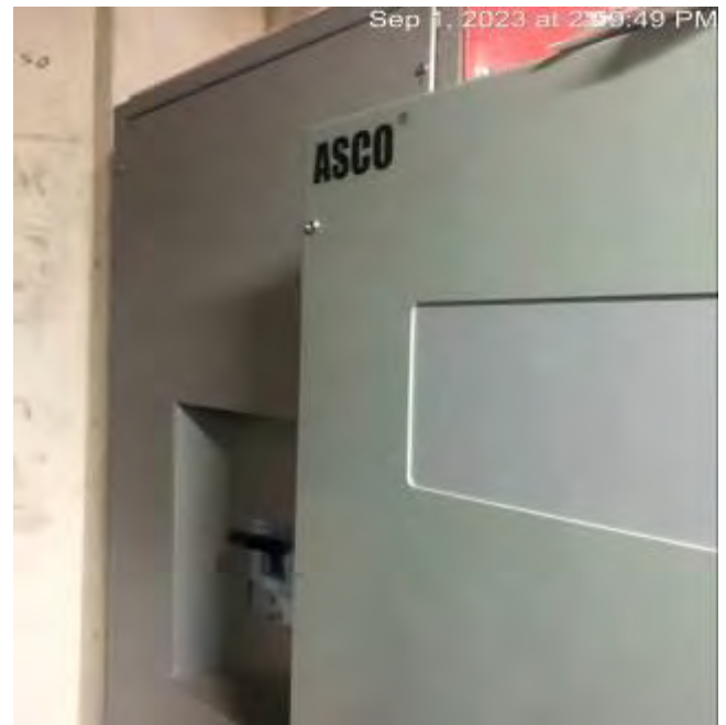
Emergency Board with ASCO ATS
