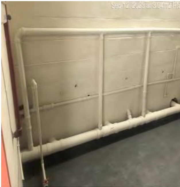
Typical Toilet Waste & Revent Lines in AHU Room
