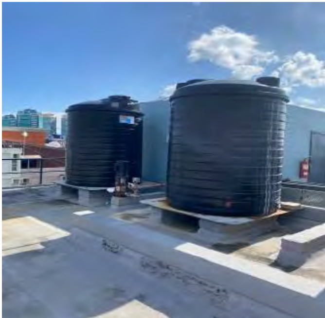
Building Potable & Fire Water Tanks on Roof Level
