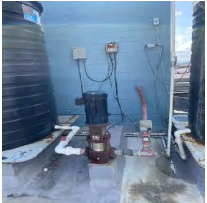
Building Potable Water & Fire Pump on Roof Level
