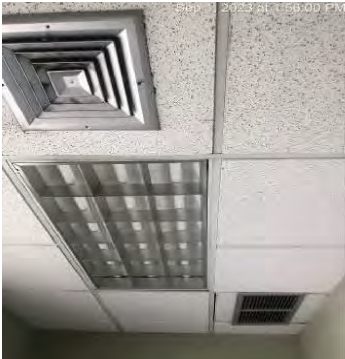
Supply Diffuser and Return Grille
