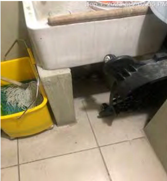
Janitor sink within Janitor room missing the required floor drain
