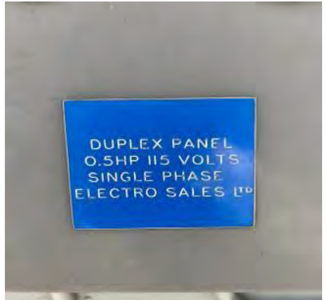
Sump pump control panel
