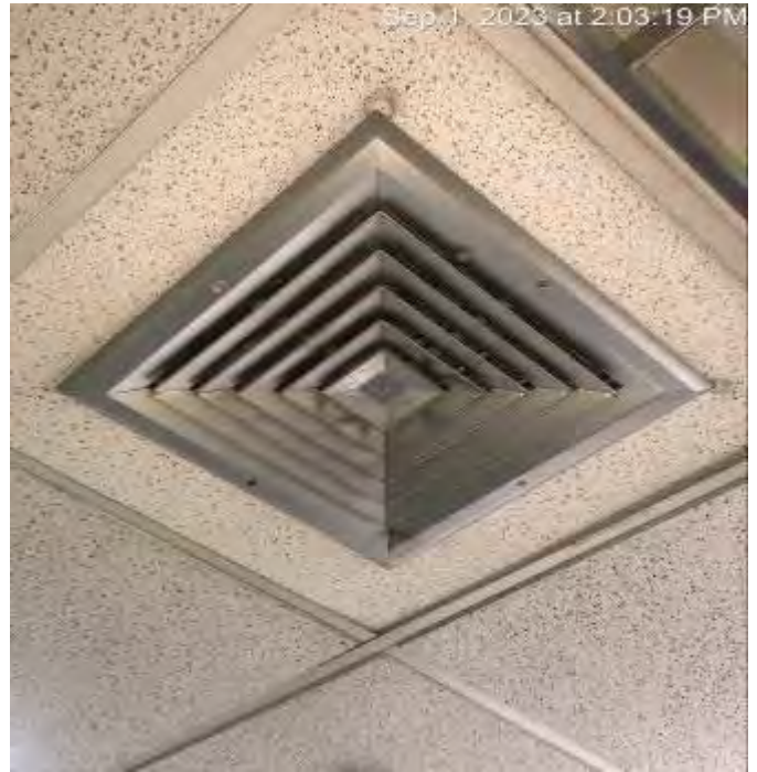
Supply Diffuser with OB damper
