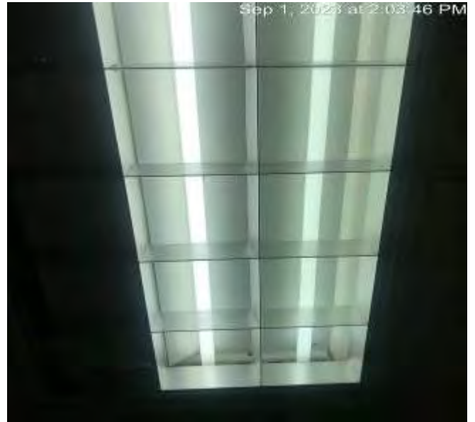
General Office 4 ft x 2 ft Light Fixture with Fluorescent Bulbs
