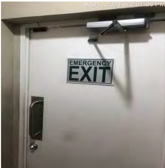
Emergency Exit door with intrusion alarm sensor
