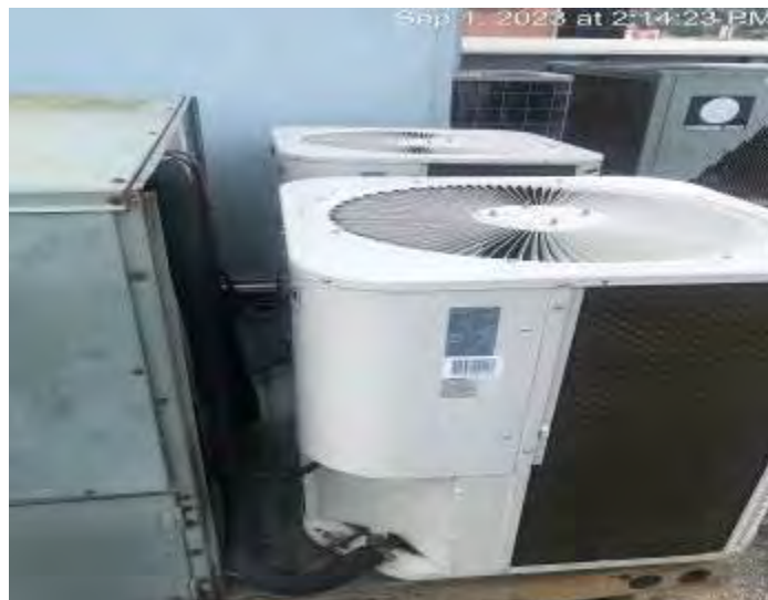
Rheem 10 Ton Package AC unit modified with (2) 5 Ton Split unit Condensers
