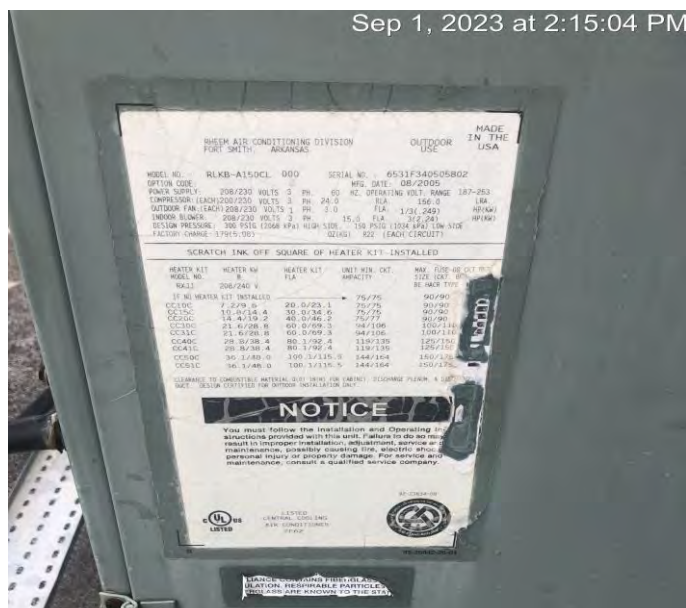
Rheem 12.5 Ton Package AC unit with manufacture date of 2005 label
