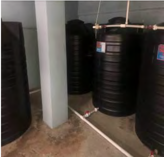
Building Fire Water Tank Farm in Basement Level
