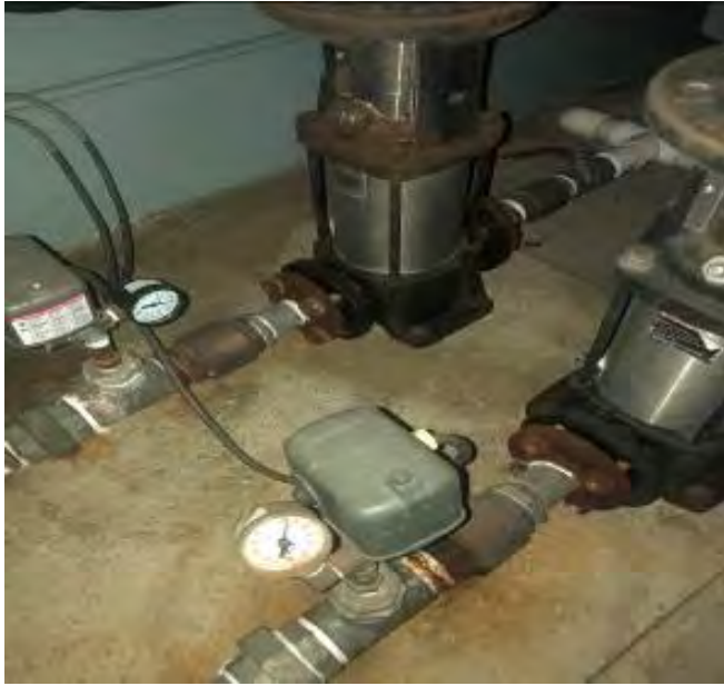
Potable & Fire Water Duplex Pump Set
