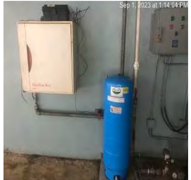
Fire Hose Reel Cabinet & Pressure Tank
