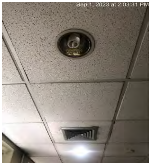
Outdated Recessed Downlight Can with fluorescent light bulb
