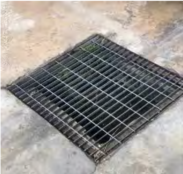
Basement drain catch pit
