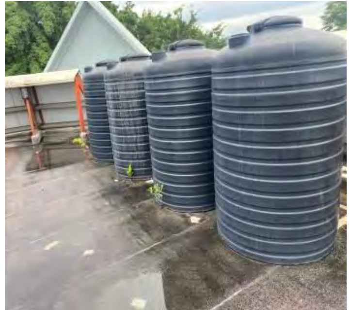
Building Potable Water Tank Farm on Roof Level
