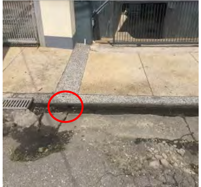
Sump Pump discharge line exit onto Lucknow Street
