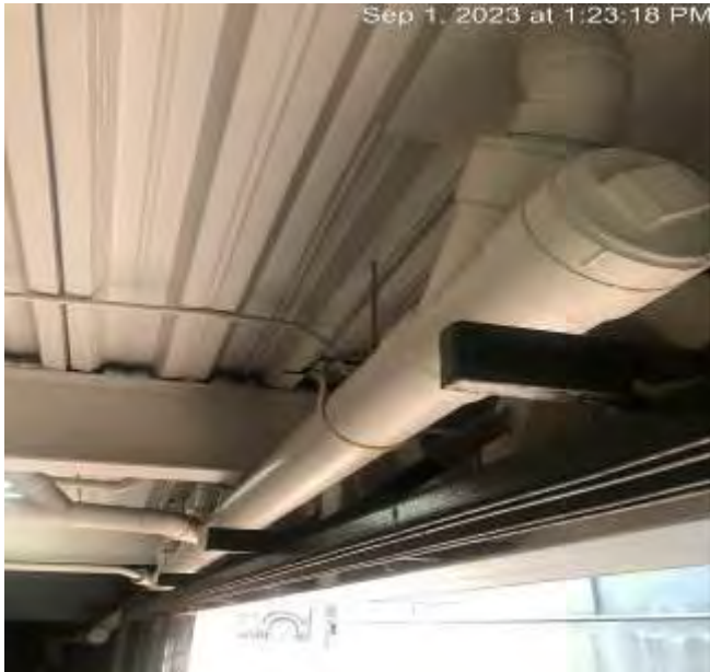
Main 6" Waste water line to sewer
