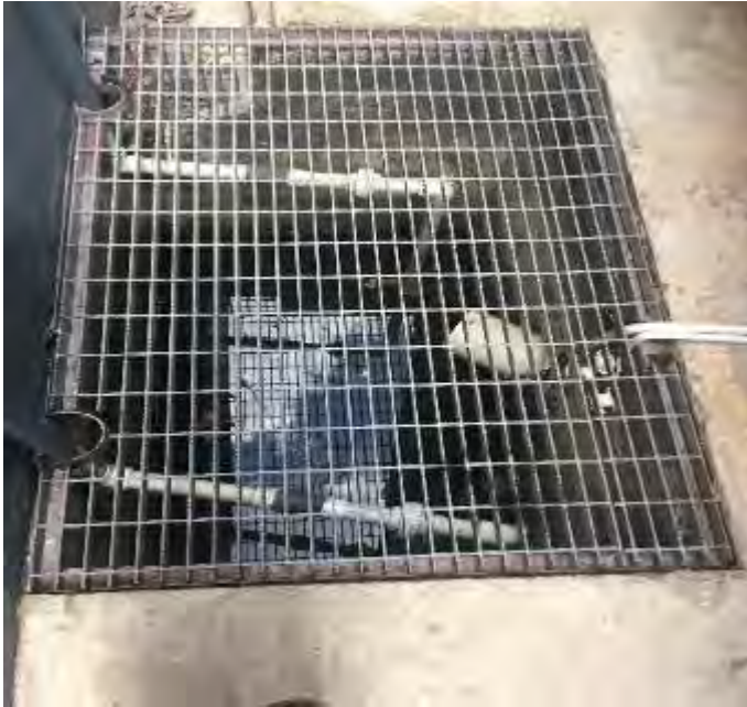
Existing Sump Pump Pit with pump and grating cover
