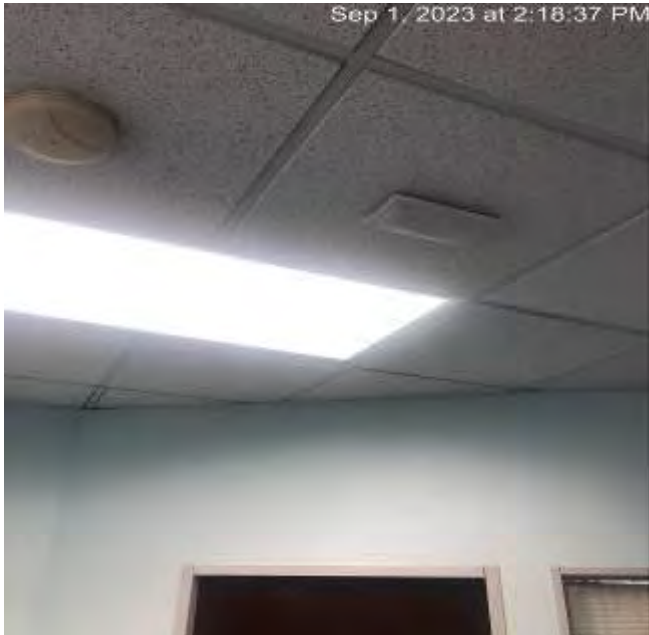
Smoke Detector and Wireless Access Point
