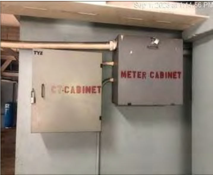
T&TEC C.T and Meter Cabinets
